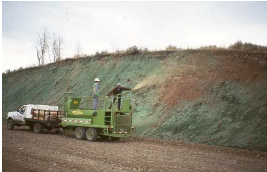
Applying a tackifier using a trailer mounted pump and hose.
