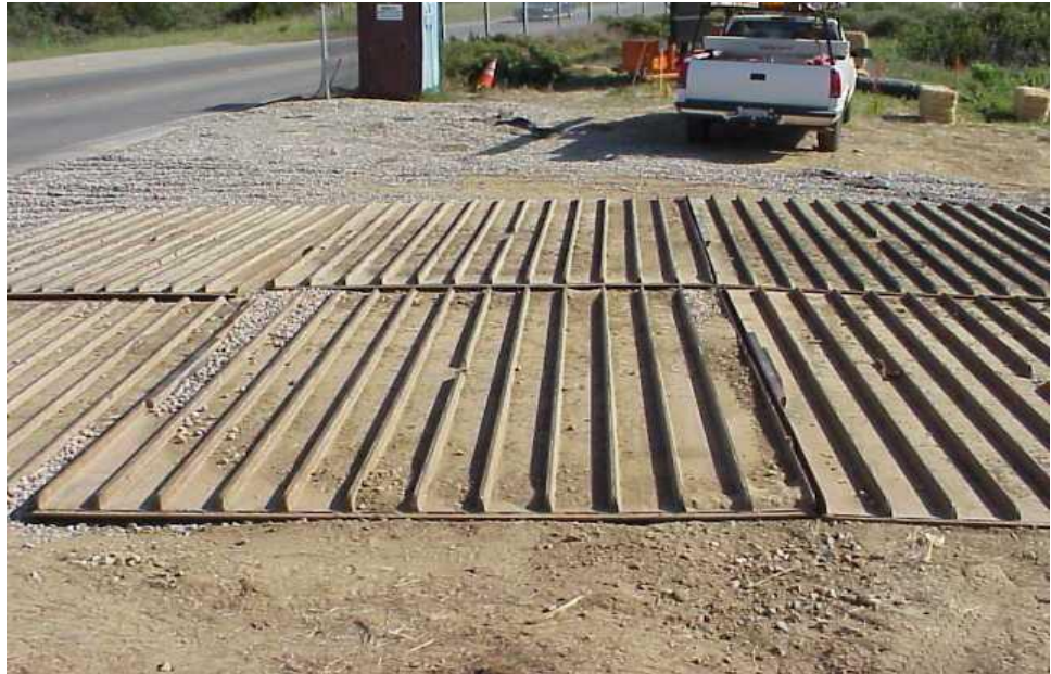
Manufactured metal plates knock dirt off vehicle tires before exiting a site.
