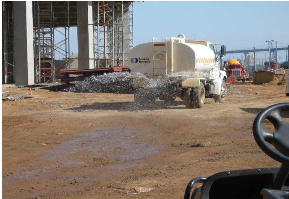
Water being applied for dust control.
