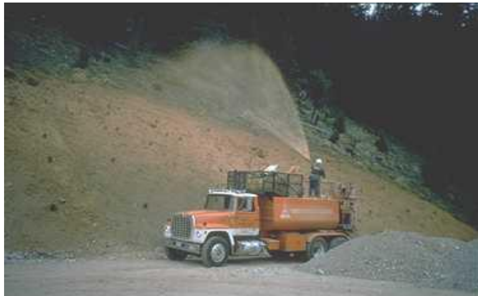
Applying hydraulic mulch.
